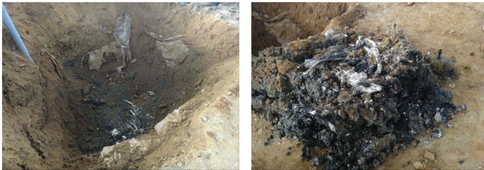
Fig. 4. Site image of demolition work.
