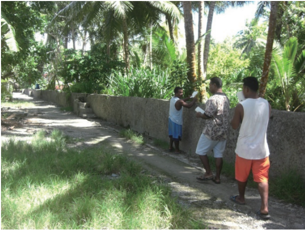
Picture 1. Seawall against high tidal wave.
