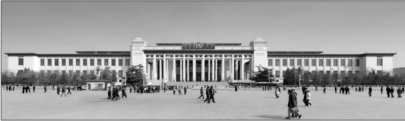
Figure 5. The restored west façade with the staggered roof of the new building, courtesy of Christian Gahl 2011
