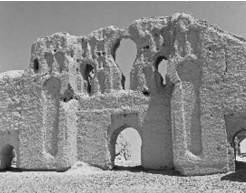
Fig. 16-1, 16-2. Central Palace (Lashkari Bazaar), Exterior and South Façade. Exterior view showing the gate and south façade with the main entrance, Bust, Afghanistan; 11th century, Ghaznavid Dynasty (photo taken in 1960). Source: https://www.archnet.org/sites/19955?media_content_id=145728
