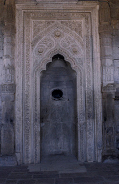
Fig. 18-1, 18-2. Seven-Arch Façade and Mihrab of the Adhai Din-ka-Jhonpra Mosque.
