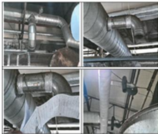
Figure 9: Air dilution case 9. Cases punished by the Won-ju Regional Environmental Office of the Ministry of Environment
