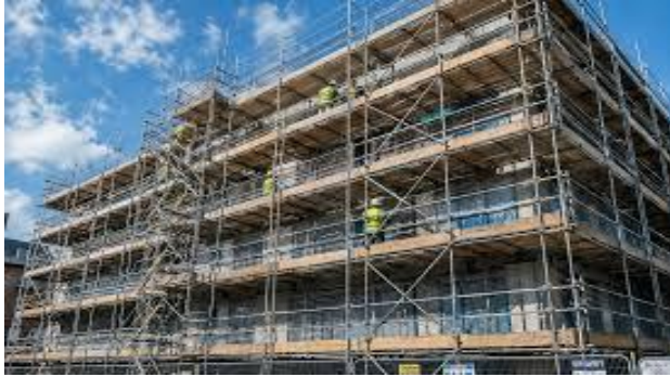
Figure 1: Safety verification and high-density installation layout of temporary scaffolding and footplates.
