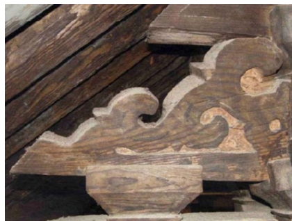
Vine-shaped Ridge Crossbeam Headpiece, Daeungjeon Hall of Sudeoksa Temple (Korea Heritage Service 2005b, 34)
