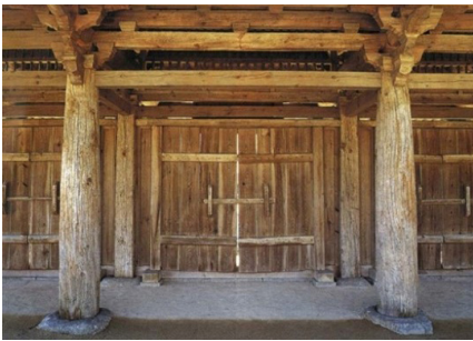
Entasis Columns, Sammun Gate of Imyeongwan Guesthouse in Gangneung (Korea Heritage Service 2004, 15)
