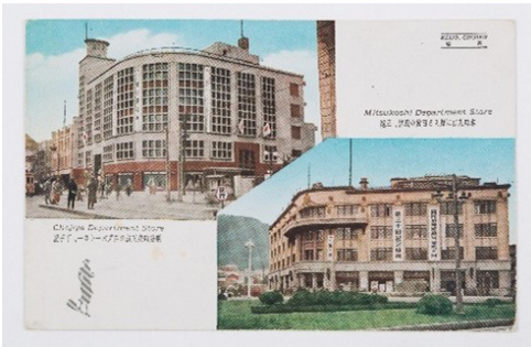
Figure 7. The Panopticon Structure of the Seodaemun Prison, a Symbol of Colonial Oppression, and the Department Store as a Symbol of Modernity (upper: photographed by the author; lower: a postcard from the Japanese colonial period [National Museum of Korea eMuseum])
