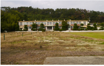
Figure 5. The Government Building Site in Okku (Sangpyeong Elementary School closed, 2016)
