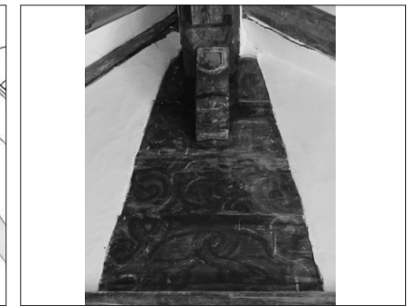
Figure 23. Horizontal Supporting Planks in Gunjajeong Pavilion, Imcheonggak House, Andong City (Photo by the Author)
