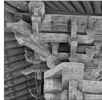
Figure 14. Frontal Corner Bracket of Daeungjeon Hall, Bongjeongsa Temple (Photo by the Author)
