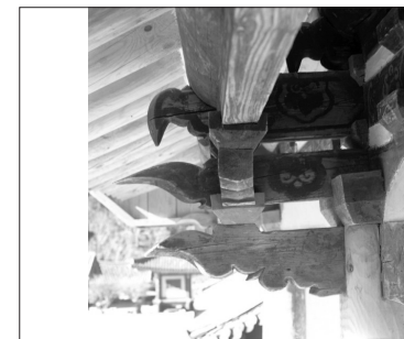
Figure 12. Bracket Set in Hasadang Hall, Songgwangsa Temple, Suncheon City
