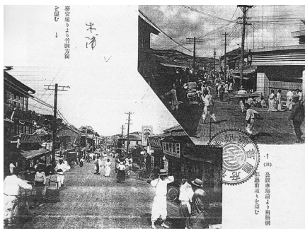
Figure 25. A View from the Market Place (upper right) and a View from Muan Street (lower left)
